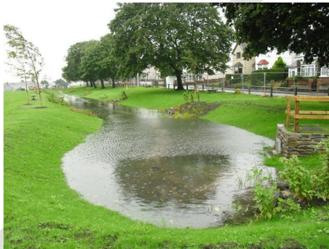
Drainage swale
